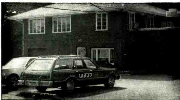
Outside view shows general character of garage converted into broadcast plant. FM antenna is on self-supporting steel monotube, seen next to left corner of building
