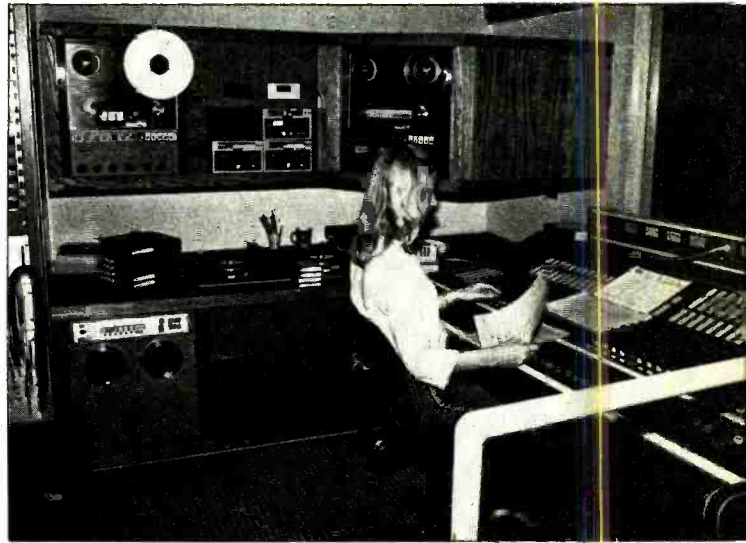
Audio control room. Audio Designs custom TV-32 audio console, Ampex ATR-700 audio tape machines, RCA cartridge tape, and timers. One timer is slaved to the directors for segment timing
